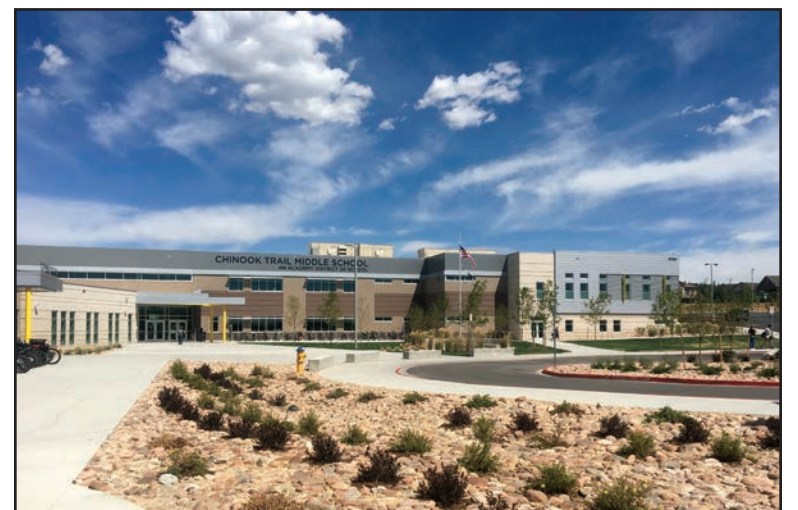
The new school incorporates sustainability and energy-efficiency design and construction standards.
